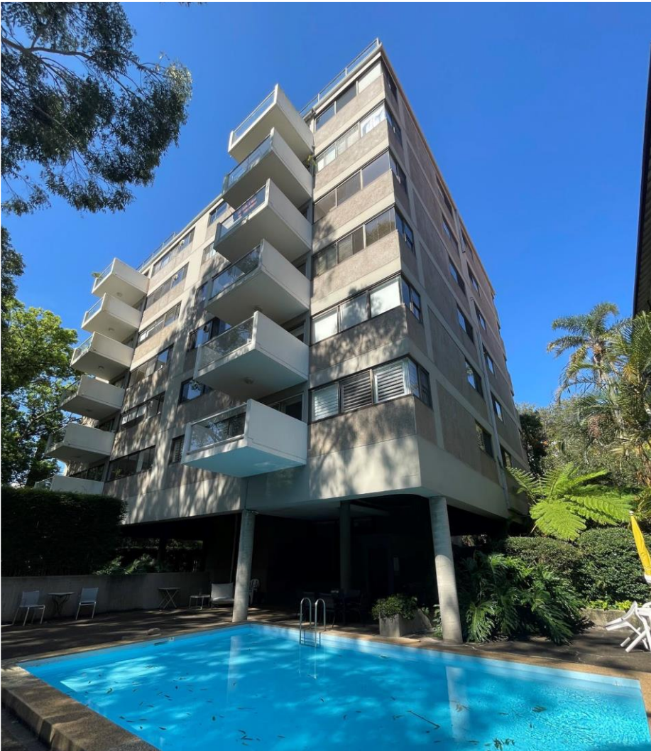
Figure 12. Rear view of 1–5 Clement Street showing pool, deep projecting balcony units and wrap around window elements to corners. Source. GML, 2024.
